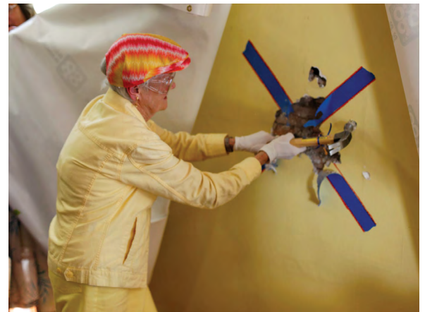
CAROL BREAKS GROUND AT SHERMAN Carol Davis Norberg attended Sherman's ground-breaking ceremony in 2012 to initiate its retrofit. ▲
